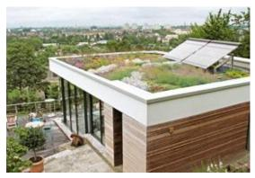
Thanks to bioplastics, the three system elements in a green roof build-up (protection mat, drainage element and filter mat) now contribute materially to climate protection, in addition to their actual environmental function.
